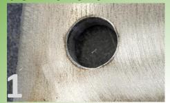
Picture 1 has been properly reworked with a powered grinder and has clean uniform edge around the diameter of the hole. Picture 2 also has clean reworked edges where laser slag was present.
